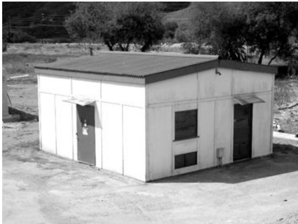
PHOTO 11. Chlorination and Booster Pumping Station/Valley Vista Building, facing southwest (30 April 2002).
