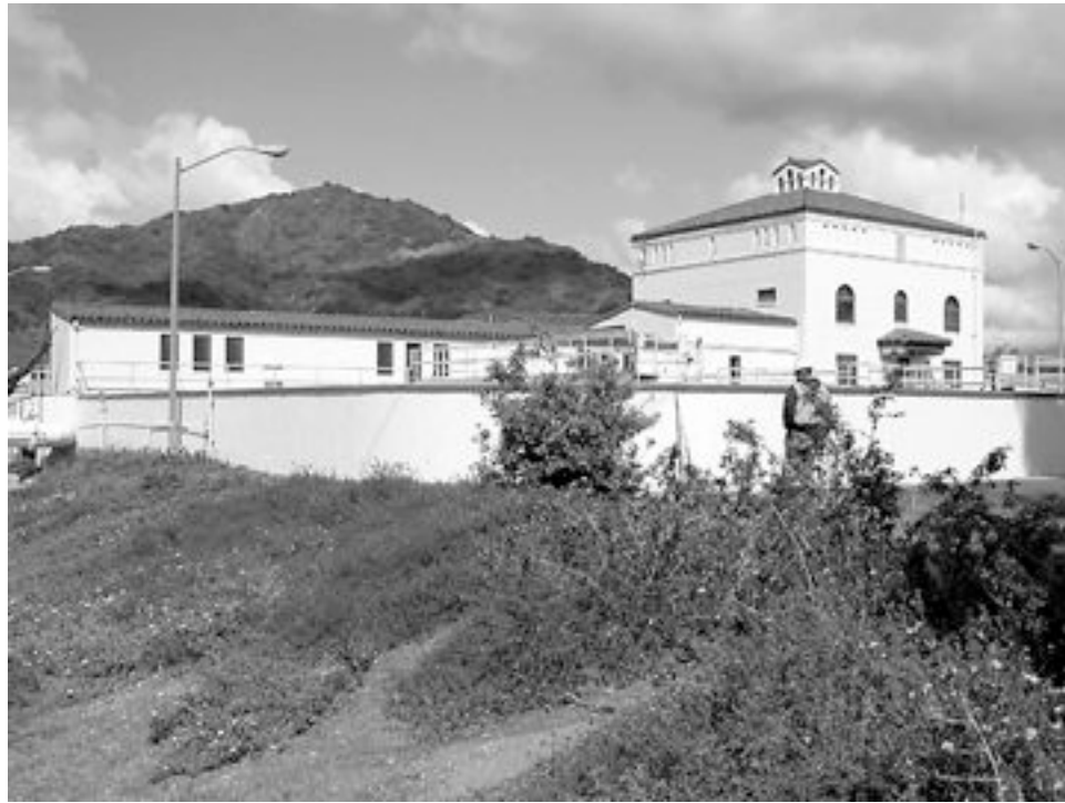
PHOTO 2. Front (eastern) elevation, Administration Building, facing northwest (30 April 2002).
