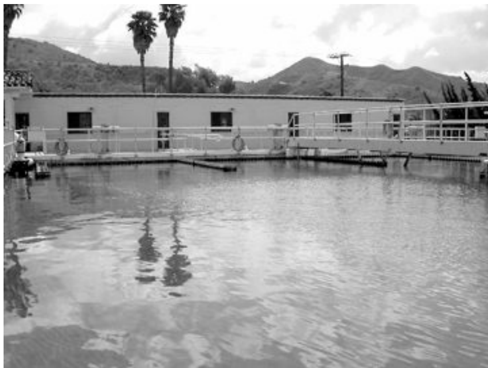
PHOTO 7. West Sedimentation Basin, facing east (30 April 2002).
