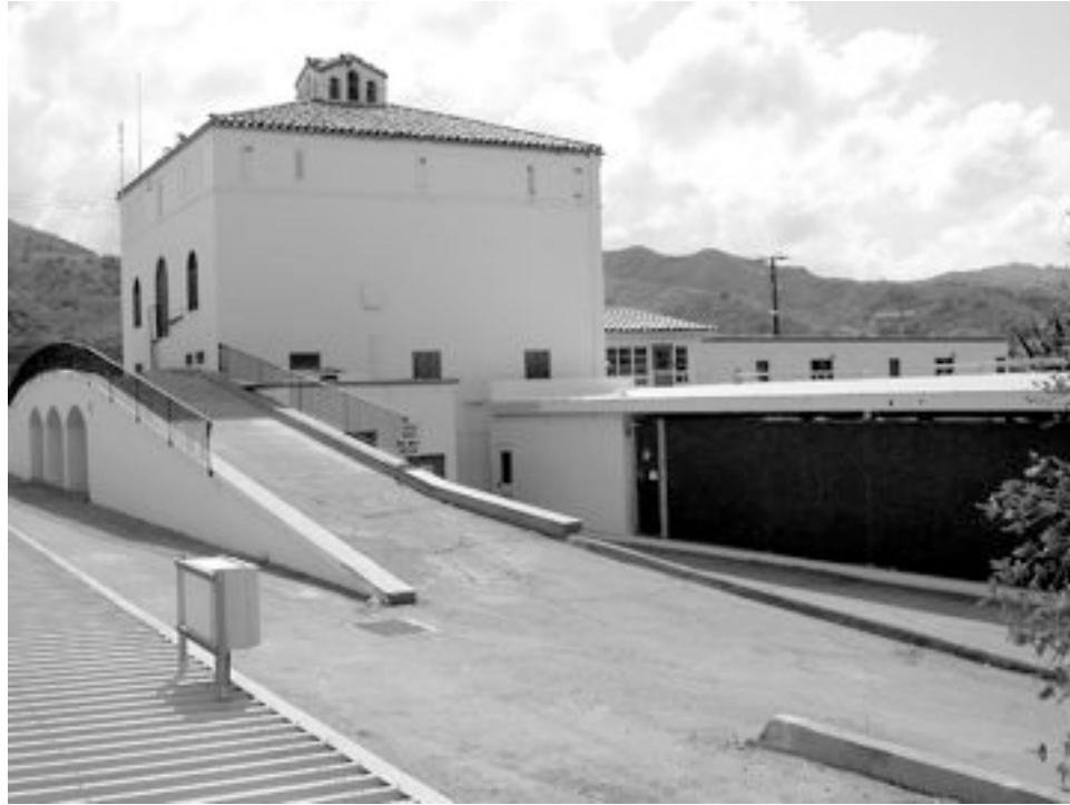
PHOTO 4. Rear (western) elevation, Administration Building, facing east (30 April 2002).
