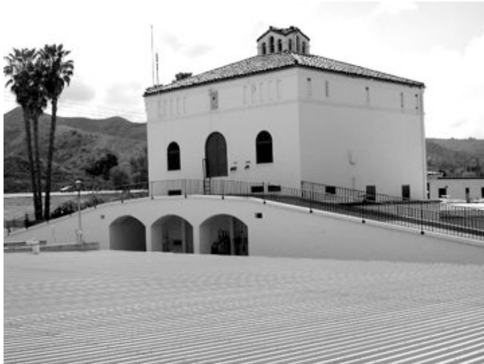
PHOTO 3. Northern and western elevation, Administration Building, Power Reservoir in foreground, facing southeast (30 April 2002).
