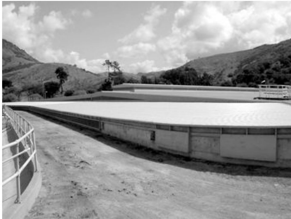
PHOTO 10. Power Reservoir, facing north (30 April 2002).
