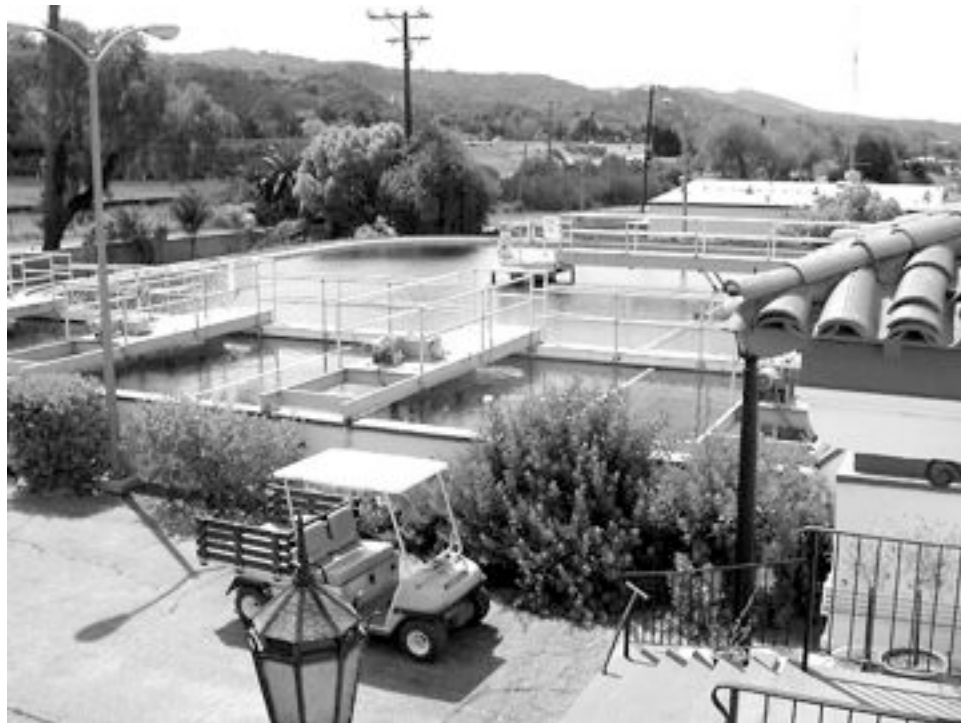
PHOTO 5. Primary Flocculator/East Sedimentation Basin, facing south (30 April 2002).
