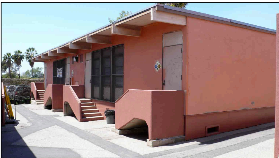
Description of Photo: (View, date, accession #) Photo 260-38. Classroom Building, eastern and northern elevations. (7 May 2007)
