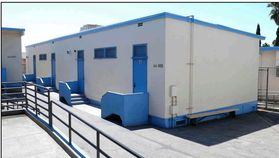
Description of Photo: (View, date, accession #) Photo 260-27. Classroom Building, northern and western elevations. (3 May 2007)
