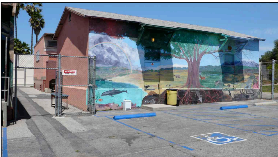
Description of Photo: (View, date, accession #) Photo 260-36. Science Building, eastern and southern elevations. (7 May 2007)
