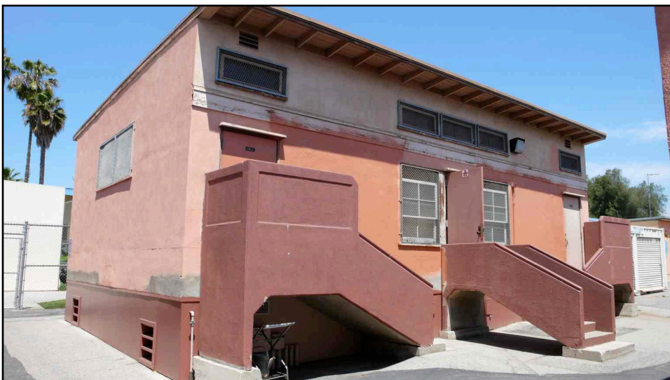
Description of Photo: (View, date, accession #) Photo 260-37. Restroom Building, eastern and southern elevations. (7 May 2007)
