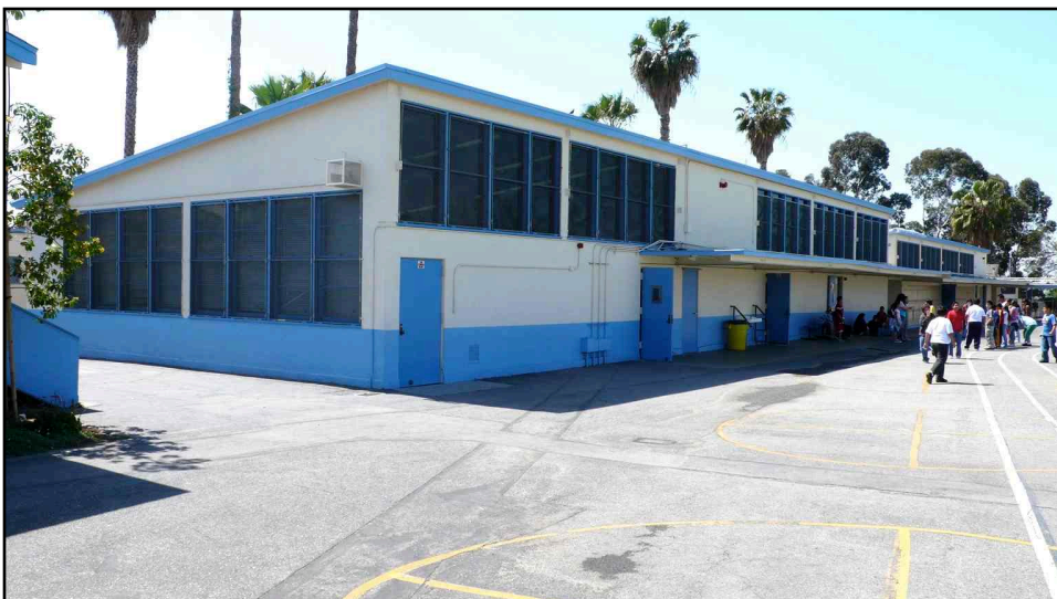
Description of Photo: (View, date, accession #) Photo 260-15. Classroom Building, western and northern elevations. (3 May 2007)
