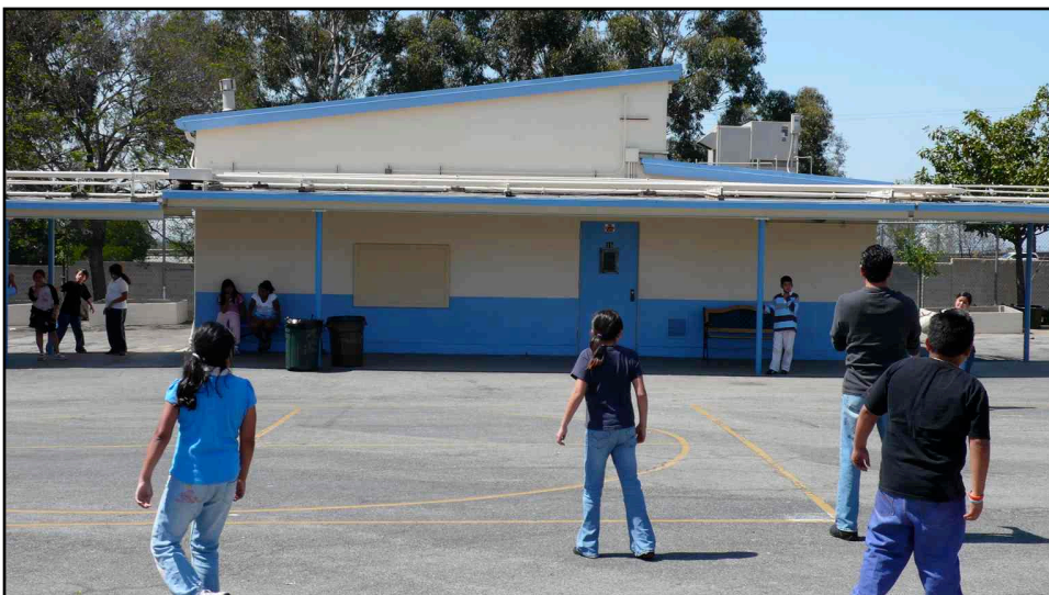
Description of Photo: (View, date, accession #) Photo 260-18. Classroom Building, northern elevation. (3 May 2007)
