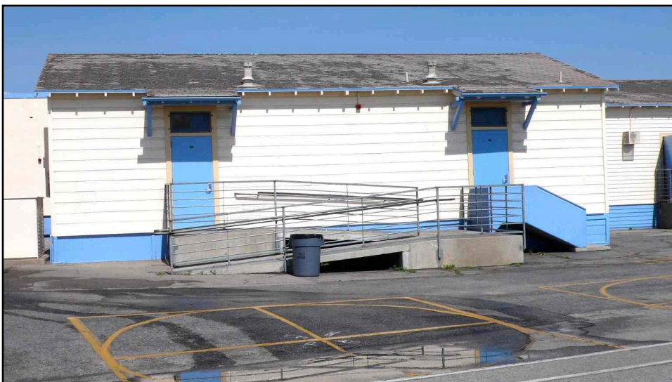
Description of Photo: (View, date, accession #) Photo 260-6. Classroom Building, eastern elevation. (7 May 2007)
