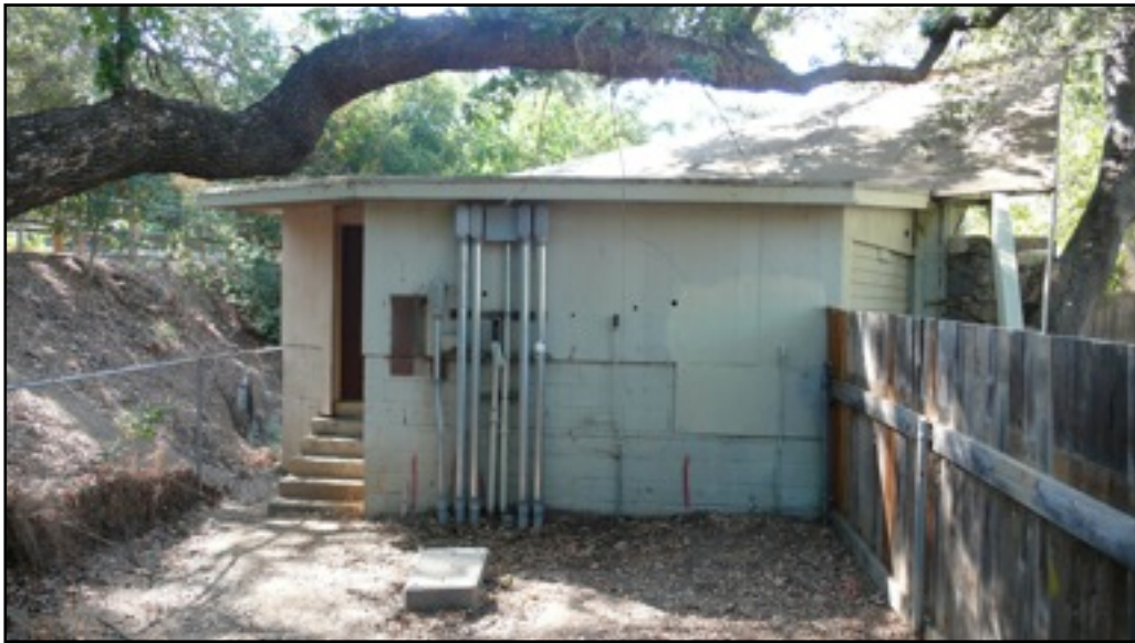
Photo 5. View of east wing of Libbey Bowl, facing west. [8 September 2008]
